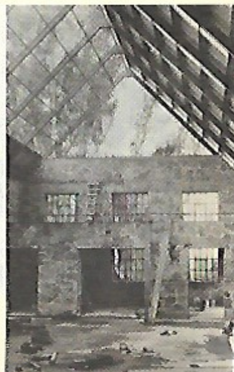
The Church of Atonement under construction
